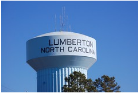
Pardue, Donald. January 29, 2011. "Water Tower. Lumberton, Robeson County, North Carolina."
