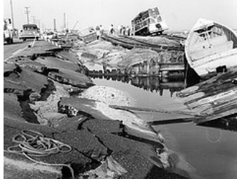
Damage from a 1960 NC hurricane. Image courtesy of the State
