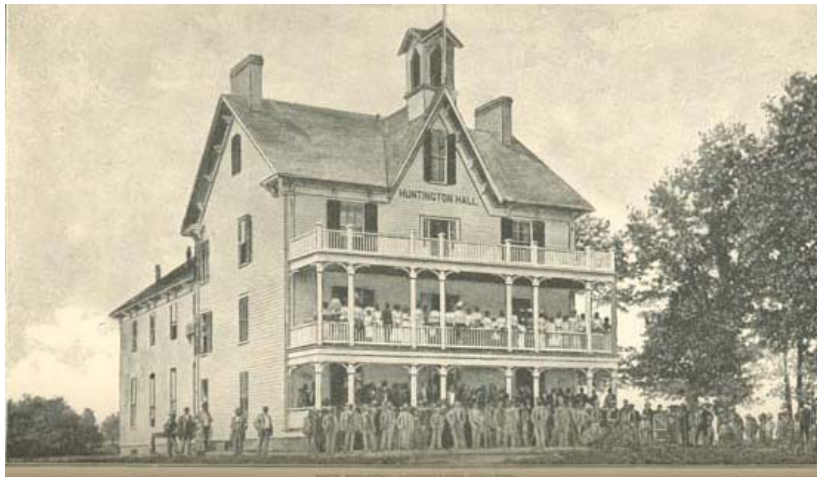
Main Building- Livingtone College, 1888. Image courtesy of DocSouth, UNC Libraries.
