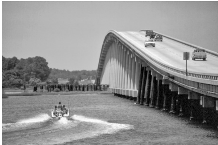
Cameron Langston Bridge over the Intracoastal Waterway on N.C. 58, connecting Cape Carteret and Emerald Isle. Photograph by Charles E. Jones. North Carolina Department of
