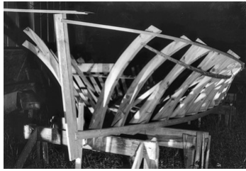
Boat in the early stages of construction at the Lewis Brothers boat works on Harkers Island, 1992. Copyright Edwin Martin, 1992. North Carolina Collection, University of North Carolina at Chapel Hill Library.
