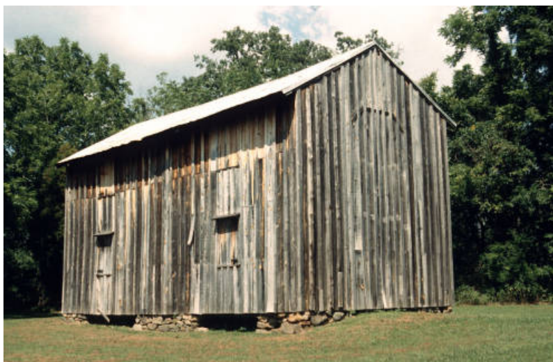
Contemporary photograph of a dwelling of enslaved persons at the Stagville Historic Site in Durham, N.C. The structure was built ca. 1851. Image from the Lauren Soth Architecture Collection at Carleton College. Used under Creative Commons license BY-NC-SA 4.0.
