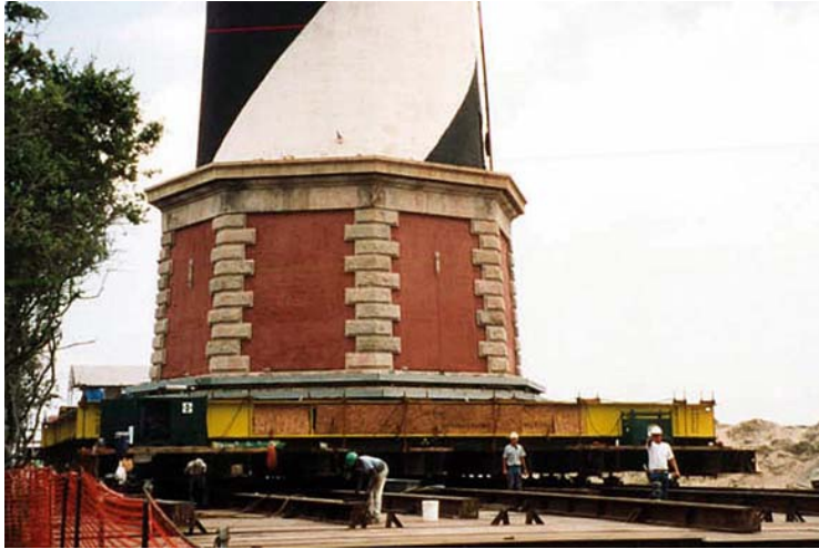
The lighthouse on tracks during its relocation.
