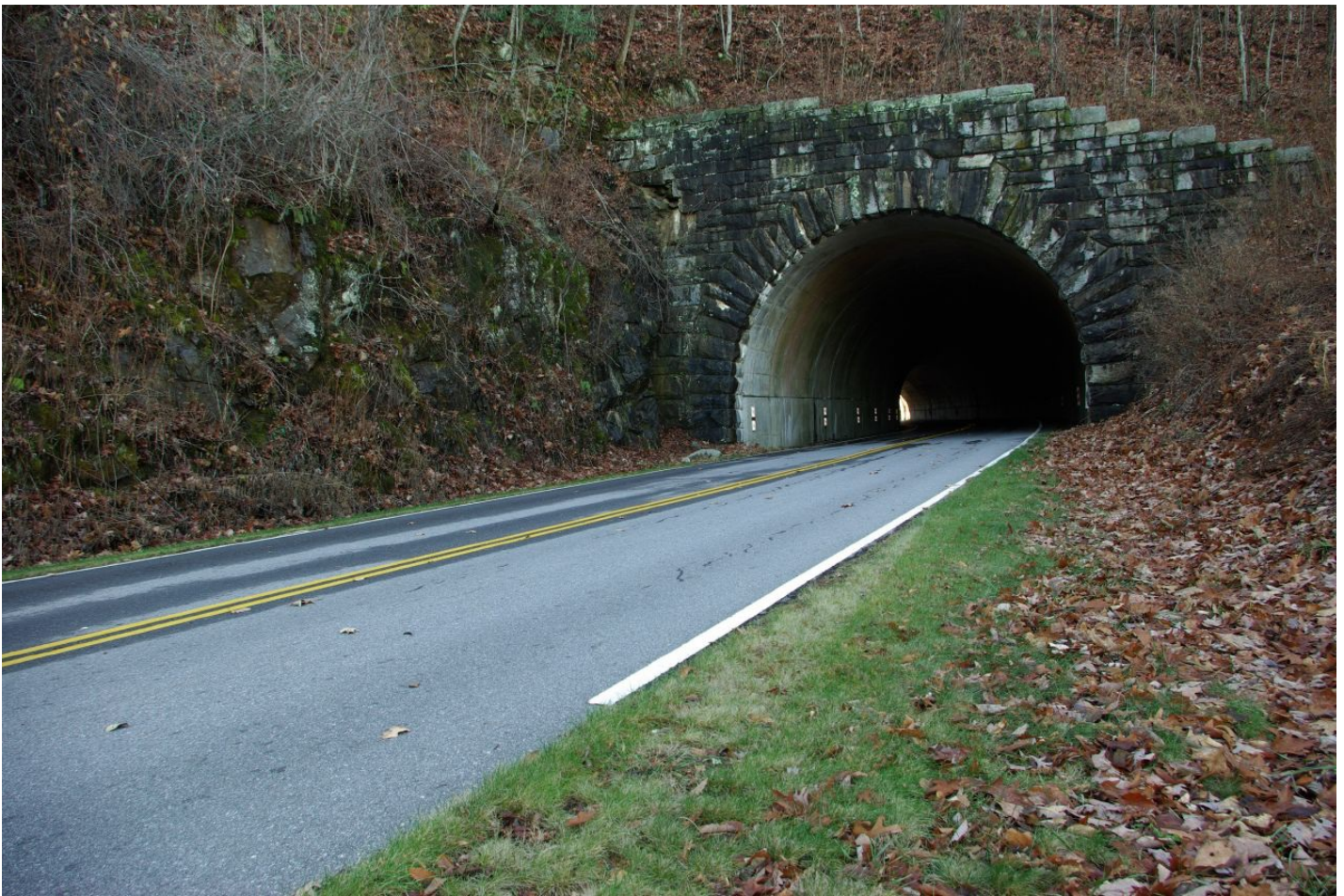
[4] The Young Pisgah Ridge Tunnel in Buncombe County is one of twenty-seven tunnels along the Blue Ridge Parkway.
