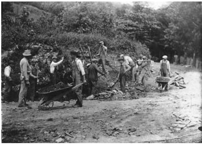
Men with shovels and wheelbarrows in a work program in Watauga County, North Carolina.
