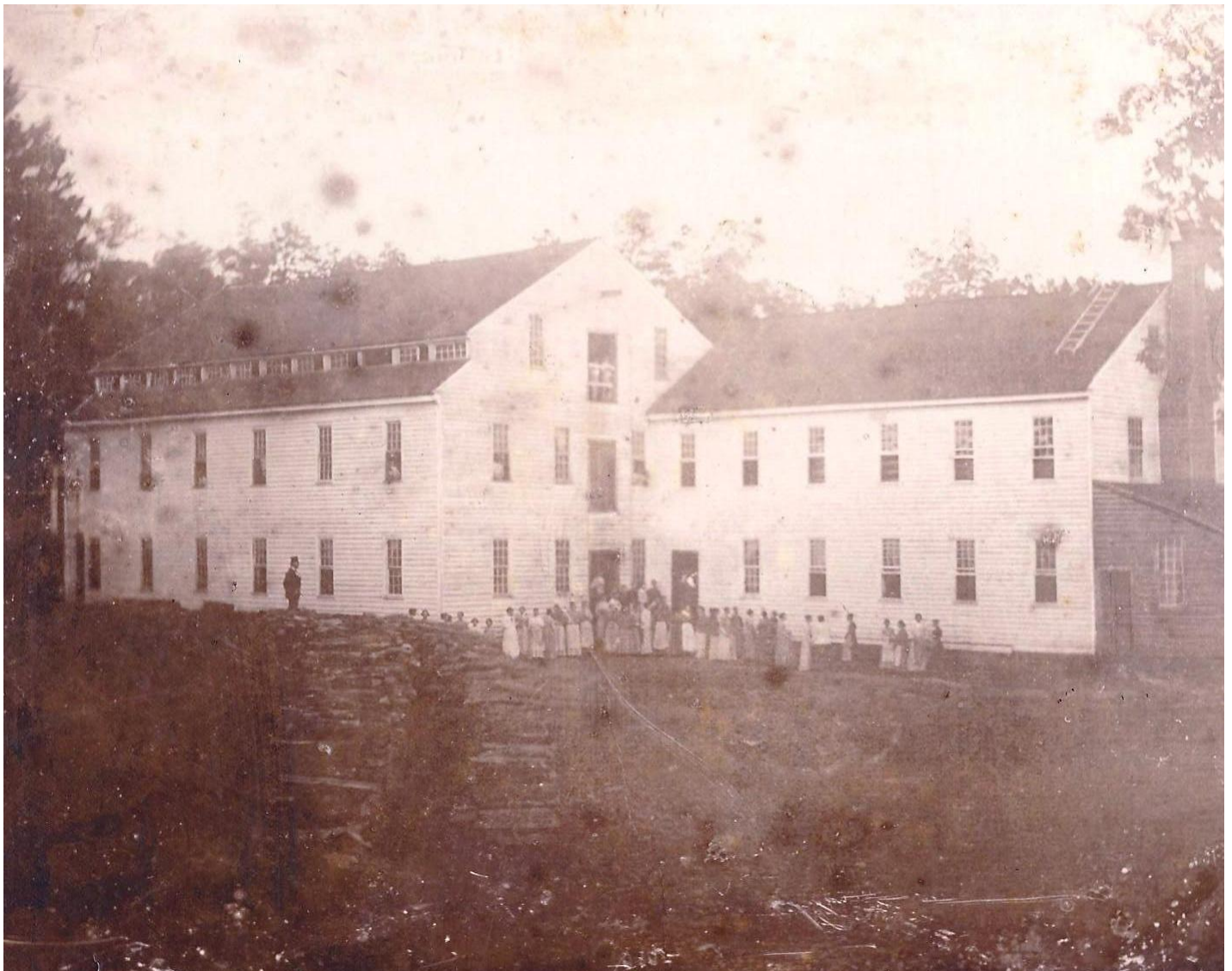
[16] This photograph of Alamance Cotton Mill and workers was taken in 1837 shortly after its construction.
