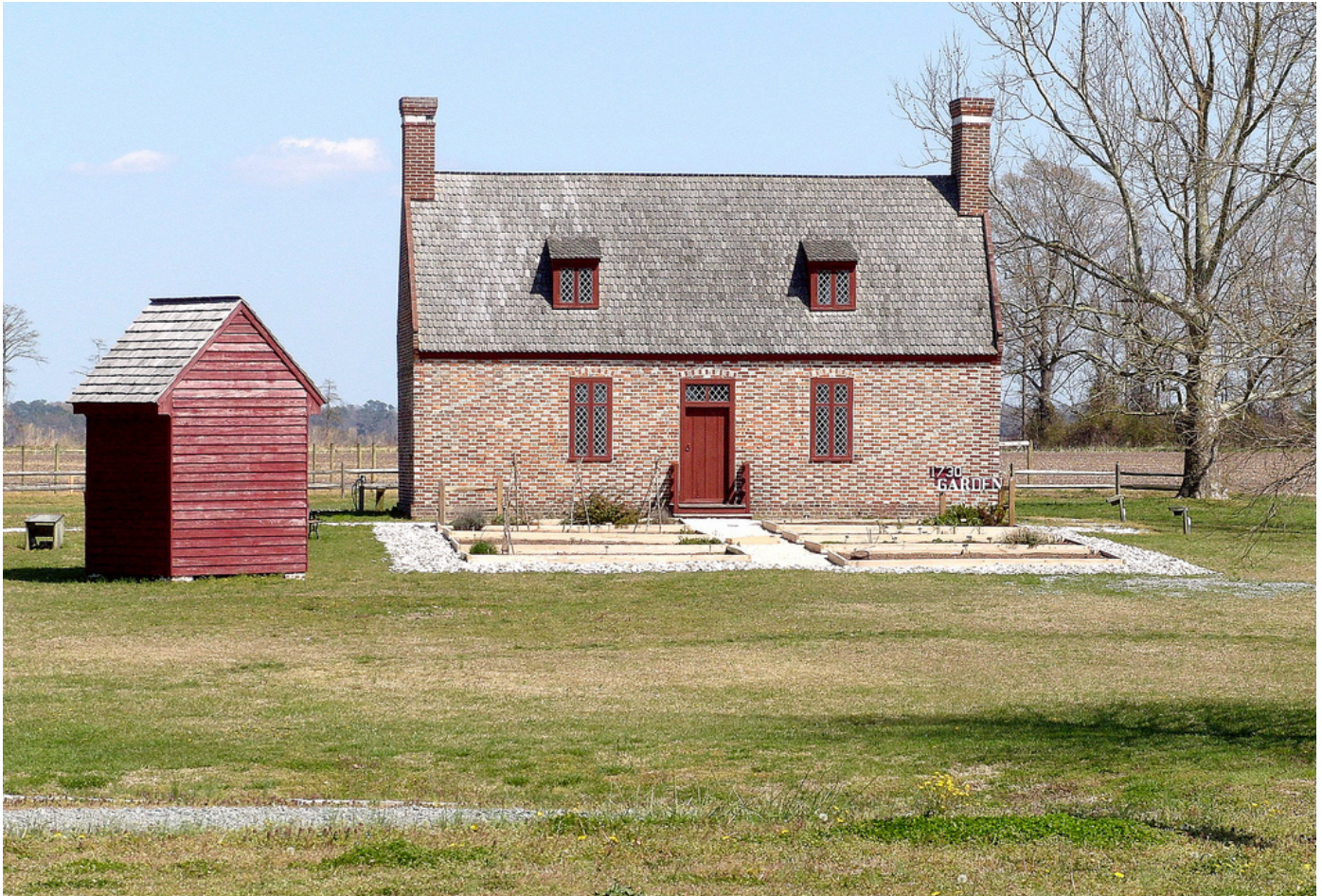
Built by Quaker farmer Abraham Sanders in 1730, the Newbold White House in Hertford is the oldest brick home in North Carolina.
