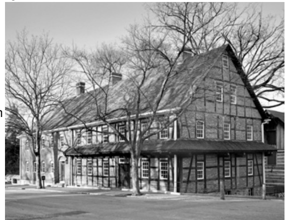
Single Brothers House at Old Salem, restored in 1964 to its 1769 condition (brick addition, 1786). Photograph by Tim Buchman. Courtesy of Preservation North Carolina.
