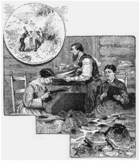
This engraving from an 1880 issue of Harper's New Monthly Magazine shows mica being mined, split, and cut near Waynesville. The accompanying text noted that the "flakes are cut in oblong squares by enormous shears, packed, and sent north. Heaps of broken wafer-like waste sheets littered the whole side of the mountain, sparkling like silver in the sun." North Carolina Collection, University of North
